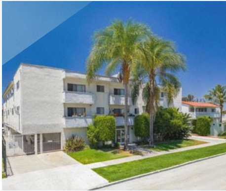
1041 S Corning Street Los Angeles, CA 90035
